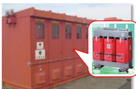
High-efficiency transformers are used in power distribution units for airport lighting systems
