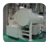
Inverter-controlled turbo chiller
