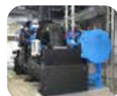
Inverter-controlled turbo chiller
