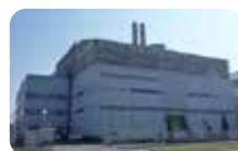
Heat supply plant
