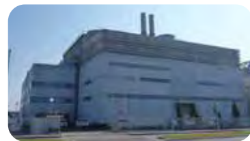
KHC Heat supply plant
