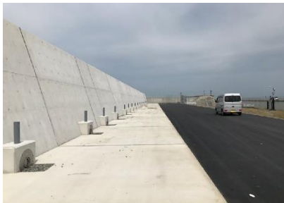
護岸の高上げ
