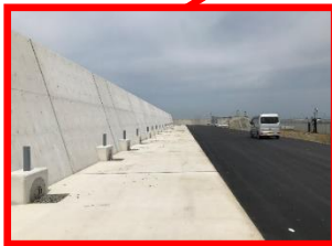
護岸の高上げ
