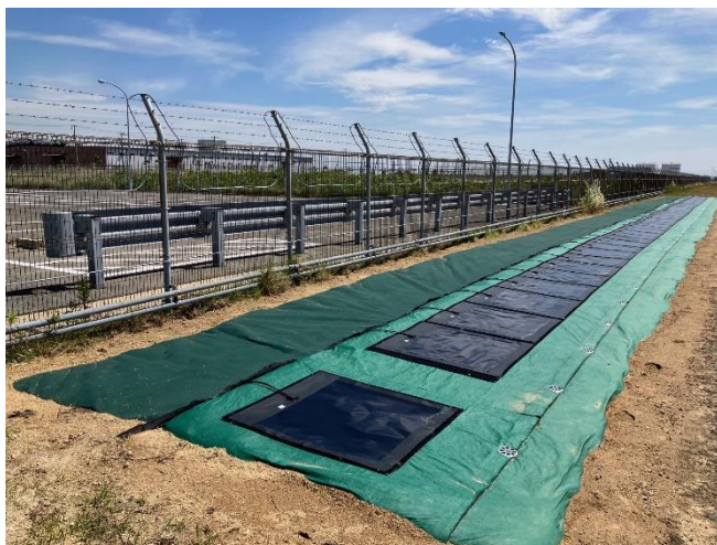
Installation of perovskite solar cells
