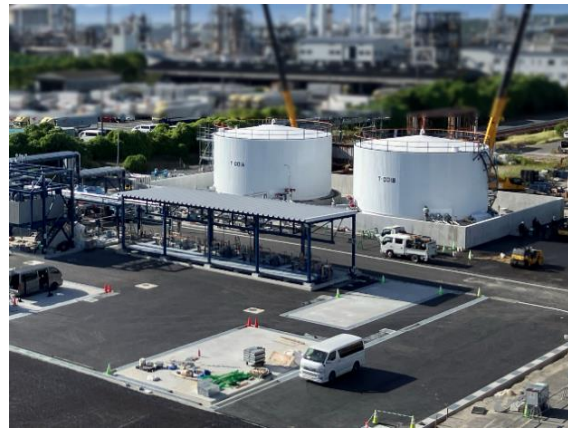
Facility for receiving waste cooking oil as SAF raw material (at Cosmo Oil Sakai Refinery)
