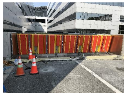
Installation of large scale water cut off barriers
