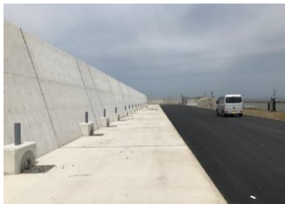
Raising of seawalls
