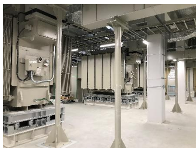
Relocation of electrical facilities above ground
