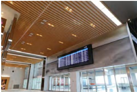
LED installation in terminal buildings
