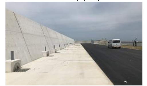
Completion of disaster resilience enhancement work (KIX)
