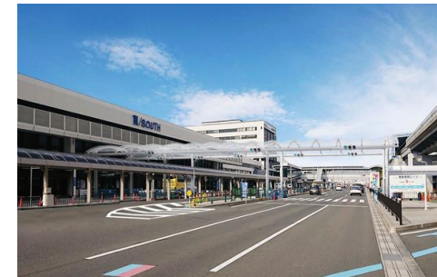
Crosswalk canopy (ITAMI)
