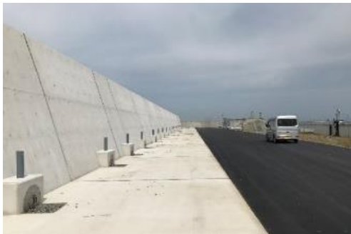
Raising of seawalls
