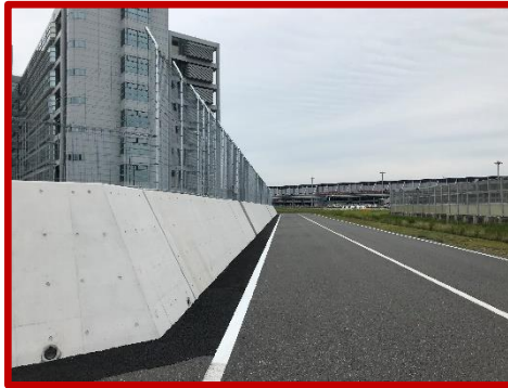
Raising and extension of cut-off walls (concrete walls)
