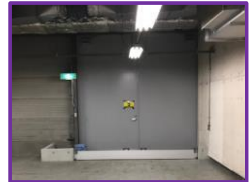
Installation of watertight doors
