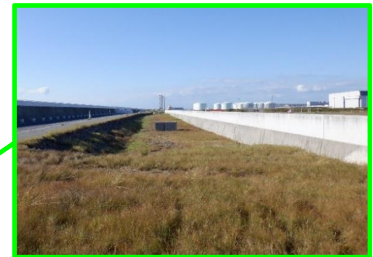
Raising of south cut-off wall
