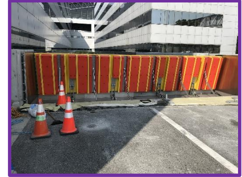
Installation of large water barriers
