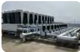
Air-cooled heat pump chillers
