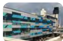
Light-blocking panels on the exterior wall of the terminal building
