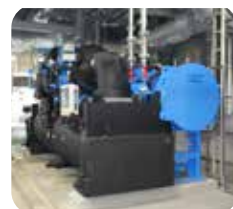
Inverter-controlled turbo chiller
