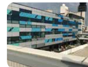
Light-blocking panels on the exterior wall of the terminal building
