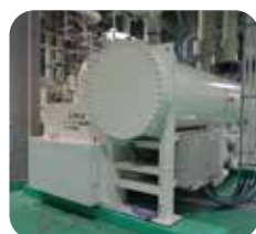
Inverter-controlled turbo chiller
