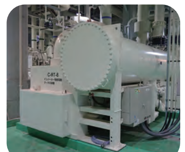
Inverter-controlled turbo chiller (KIX)
