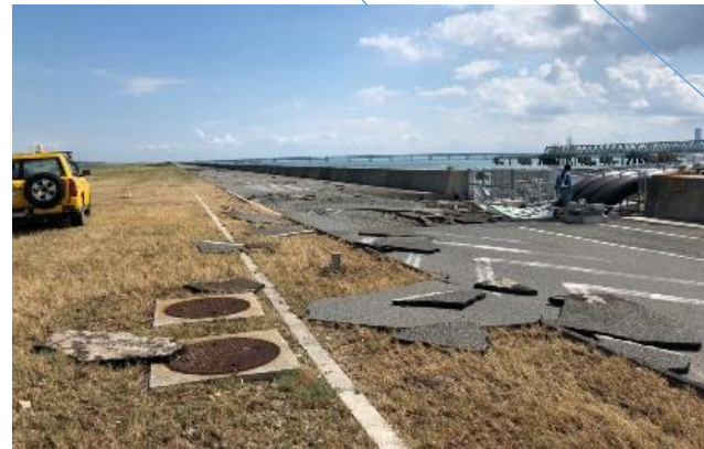
Perimeter road ripped off
