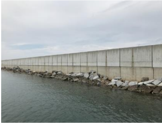
Displaced armour stone
