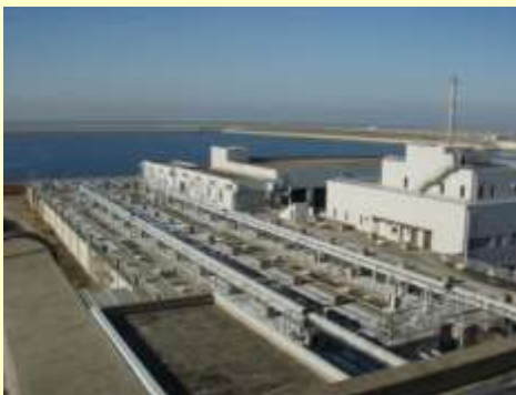
Wastewater treatment plant
