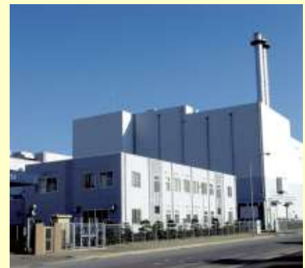
Incineration plant (Clean Center)
