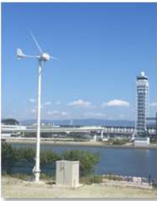
Small wind turbine generates electricity
