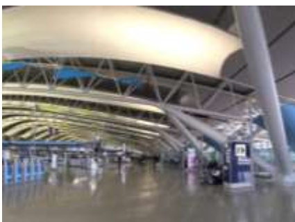
New LED lighting in Terminal 1
