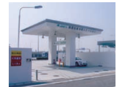
Hydrogen service station
