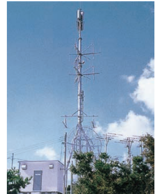
Awajimihara SHF Television Signal Relay Station This is the first time that SHF broadcasts*4 have been used in Japan in order to solve combating television signal interference caused by aircraft.
