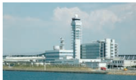
Air traffic control Emigration and Immigration management Customs Quarantine/Epidemic prevention Marine security Meteorological observatory Postal service Police service Fire defense Kansai International Airport Co., Ltd
