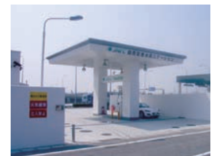
Hydrogen service station
