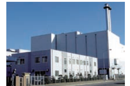
Clean Center (Incineration Plant)
