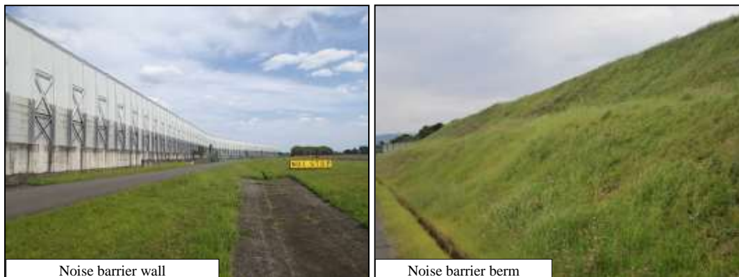
Noise barrier wall
