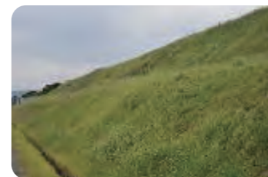
Noise protection embankments
