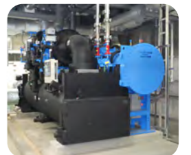
Inverter-controlled turbo chiller
