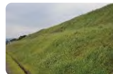
Noise protection embankments
