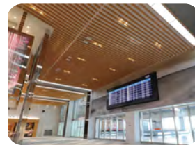
LED lighting in the terminal building (ITAMI)
