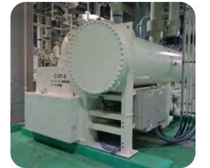
Inverter-controlled turbo chiller
