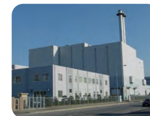
Waste Disposal Center
