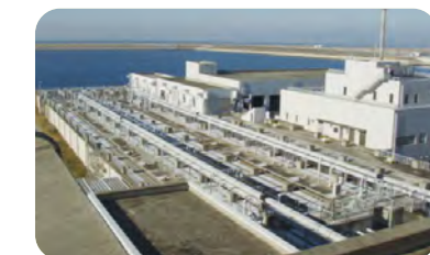
Sewage Treatment Center
