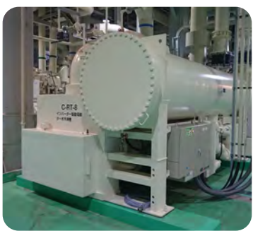
Heat-supply inverter-controlled turbo chiller
