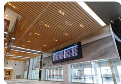
Introduce LEDs in terminal buildings
