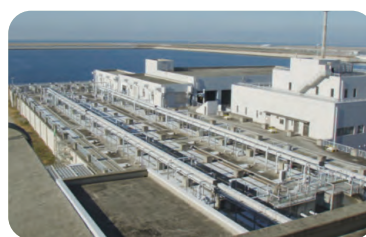
Sewage Treatment Center
