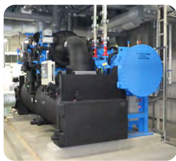
Inverter-controlled turbo chiller
