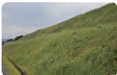
Noise protection embankments
