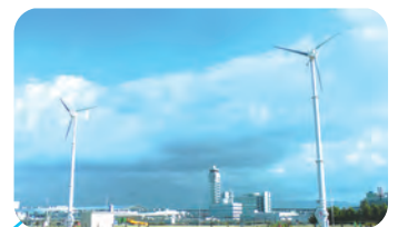
Small wind turbines
