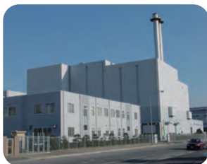
Incineration Plant (Clean Center)
