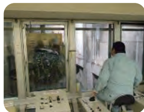
Advanced treatment of general wastewater
