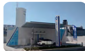
Iwatani Hydrogen Station ITAMI
